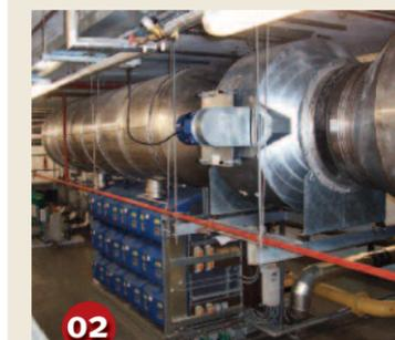
Photographs 1 and 2 (left) show the internal flue system. When the boilers are firing the fans are controlled by inverters that regulate their speed relative to the numbers of boilers firing. This was done, not only for the energy saving benefits but because the actual concentration of condensate in the system needed to be considered.
