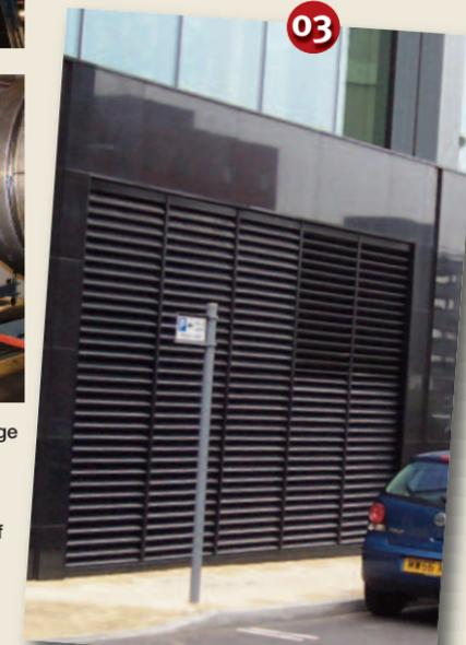
Photograph 3 (right) shows the discharge position. It should be noted planning permission had to be gained and that the requirements of IGE/UP/10 and BS6644 could not be met. As a result of this a system design verification notice had to be issued confirming the design in accordance with IGE/UP/10.
